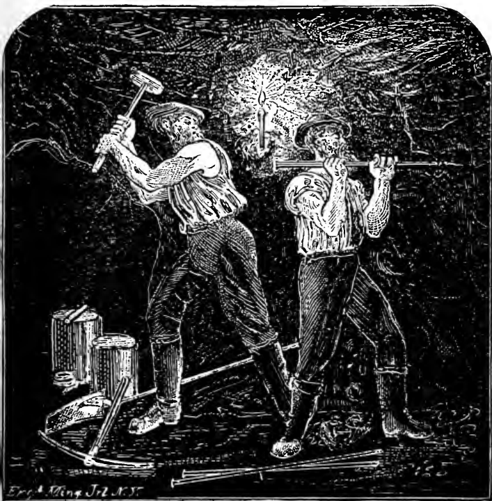
HAND DRILLING IN THE MINE.
